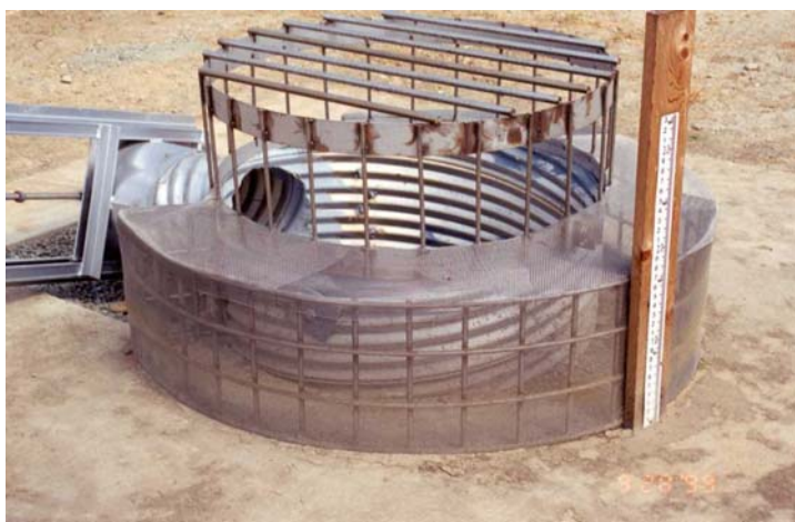
Figure 1 Example of Extended Detention Outlet Structure
